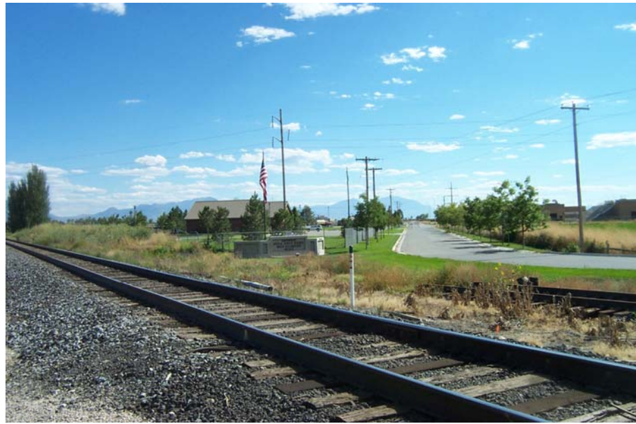
Photo 19-16. KOP 16 – Looking South toward Water Treatment Plant.
